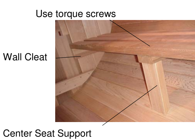
Figure 5 - Seat Installation
