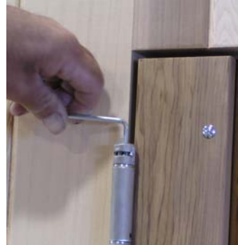
Once set pin is in place, remove wrench
